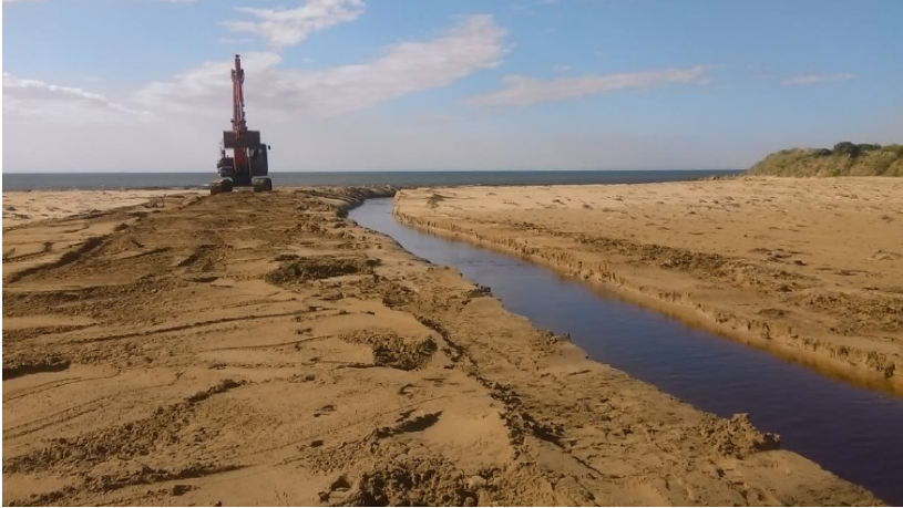
Figure 57: Mechanical opening of the Bream Creek mouth, 8 September 2016.
