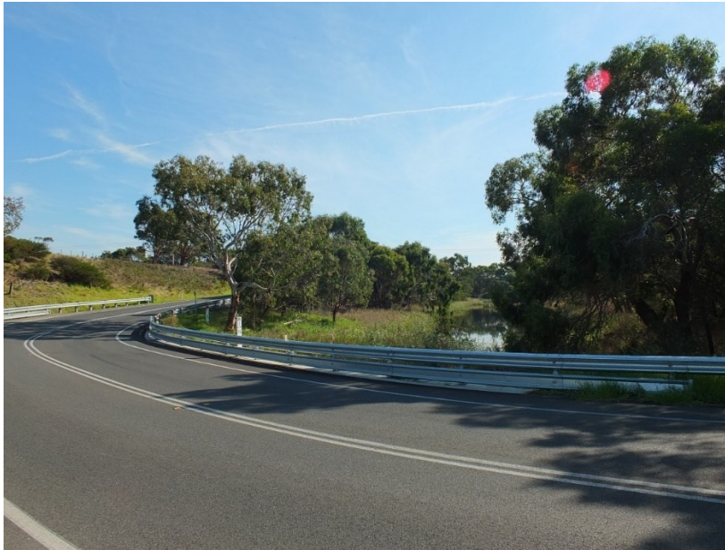
Figure 54: Culvert over Thomson's Creek, Horseshoe Bend Road, April 2022.
