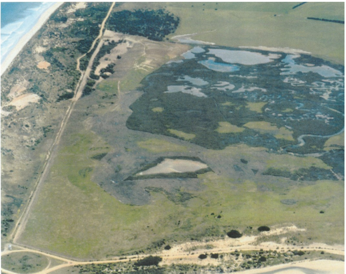
Figure 59a: Aerial view showing extent of bulldozing in the Karaaf, 1998. Source: Glenda Shomaly (with permission).
