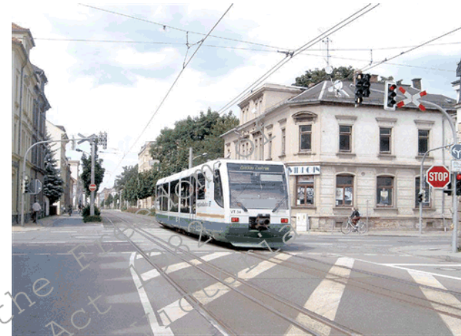
Figure 27 The Zwickau Model has main-line lightweight diesel tram-trains running through urban streets.
