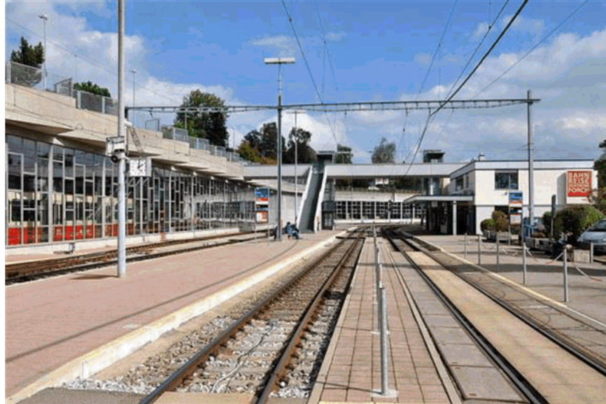
Figure 10 The station and depot at Forch
