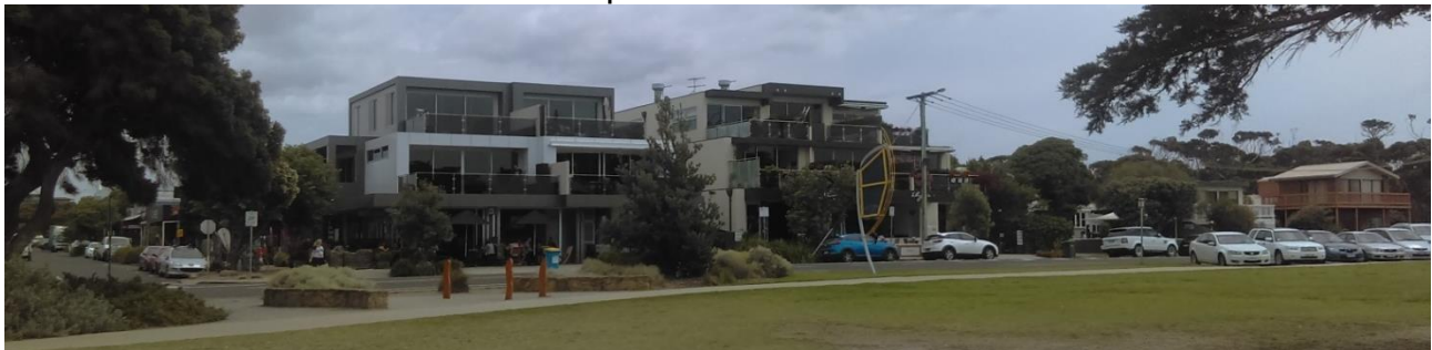
Below – view from foreshore before removal of rooftop fans
