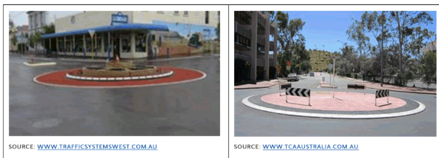
FIGURE 6: EXAMPLES OF A REMOVABLE RUBBER ROUNDABOUT
