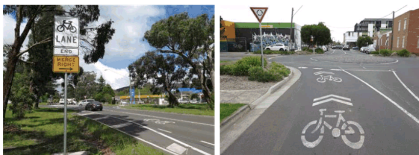
FIGURE 9: EXAMPLE OF BICYCLE TREATMENT AT A ROUNDABOUT – BICYCLE LANE TERMINATES ON THE APPROACH AND SHARROWS ARE PROVIDED IN THE TRAFFIC LANE TO INDICATE THAT CYCLISTS ARE TO MERGE AND SHARE THE TRAFFIC LANE
