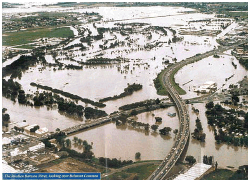
The Barwon River flooding, from Belmont Common, November 1995.
