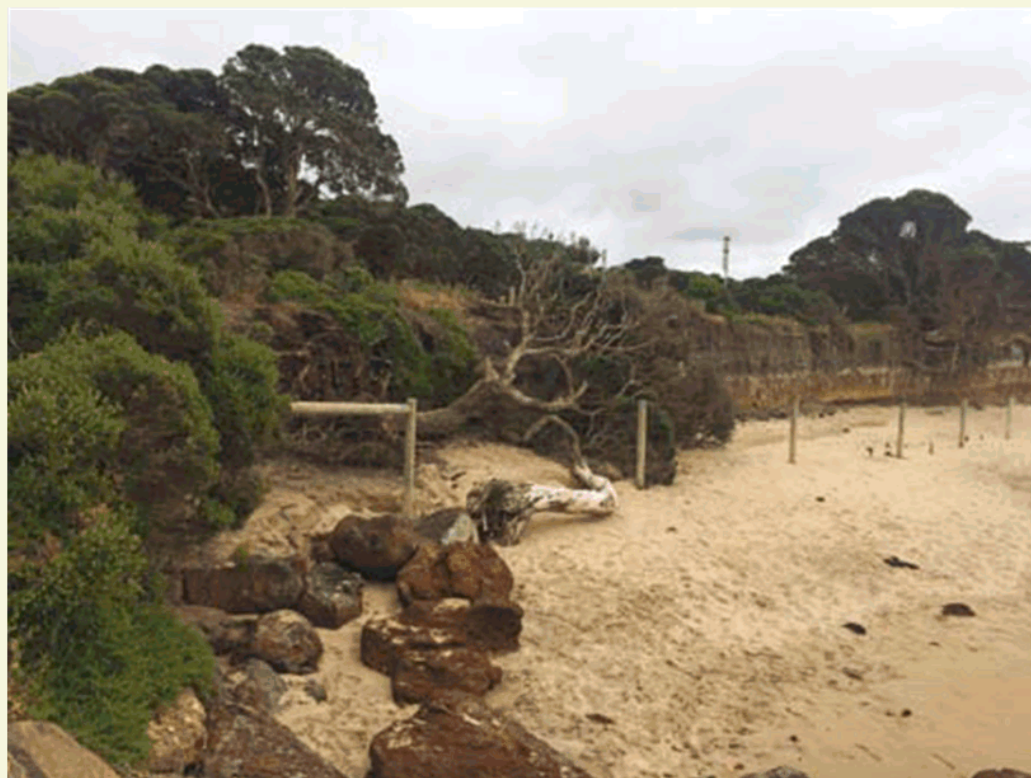
Erosion along Point Roadknight beach, Anglesea.
