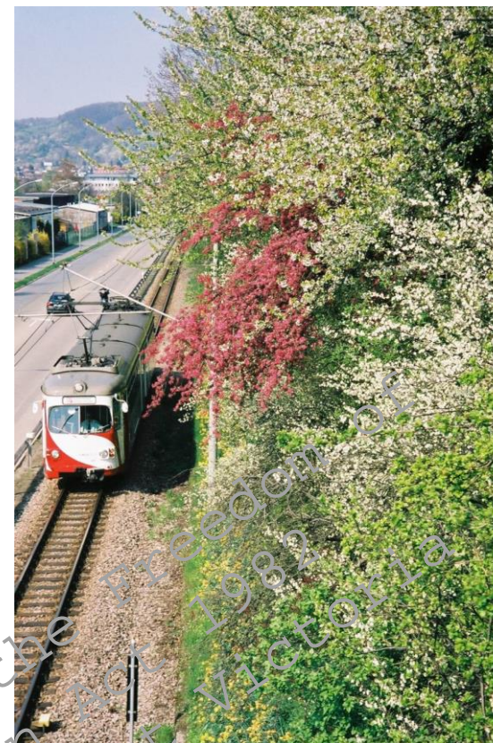
Figure 15 Roadside operations, Upper Rhine Railway
