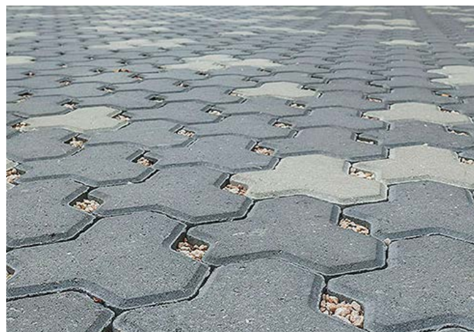
Permeable pavers Permeable paving, providing all-weather access and addressing issues associated with wash-out of gravel onto tennis courts. (Product pictured: Eco Trihex Paver, manufactured by Adbri)
