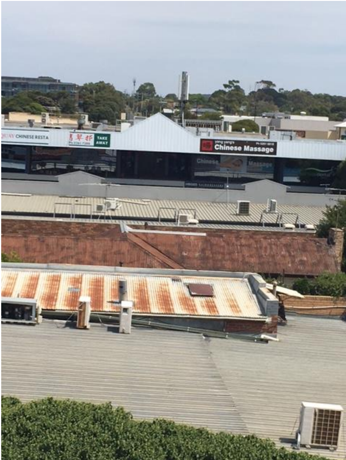
Figure E – Photo of behind the building toward Gilbert St, snapshot showing just some of the other roof mounted condensers of other properties picked up in past acoustic reports.
