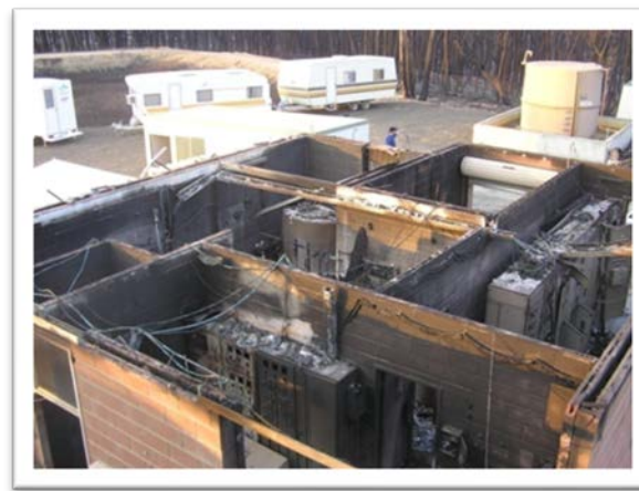
Figure 32 and Figure 33 Damage to a water pumping plant which occurred during the 2009 Black Saturday fires
