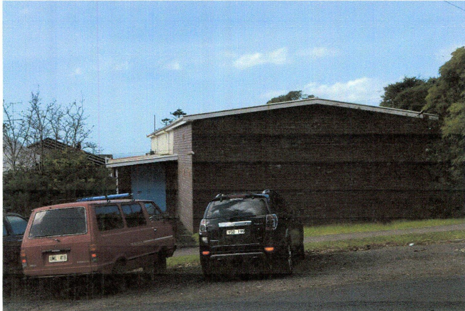
Hall to the rear of the site as seen from Smith Street.
