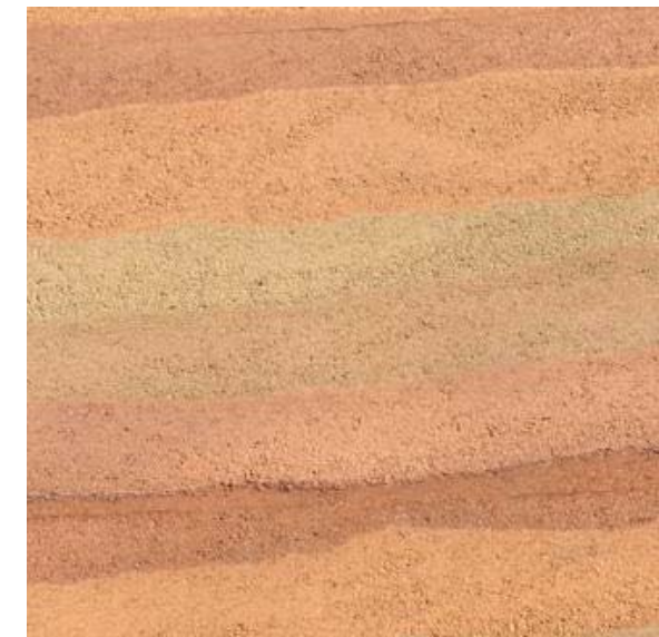
RE1 - CEMENT STABILISED RAMMED EARTH - JAROSITE CLAYS
