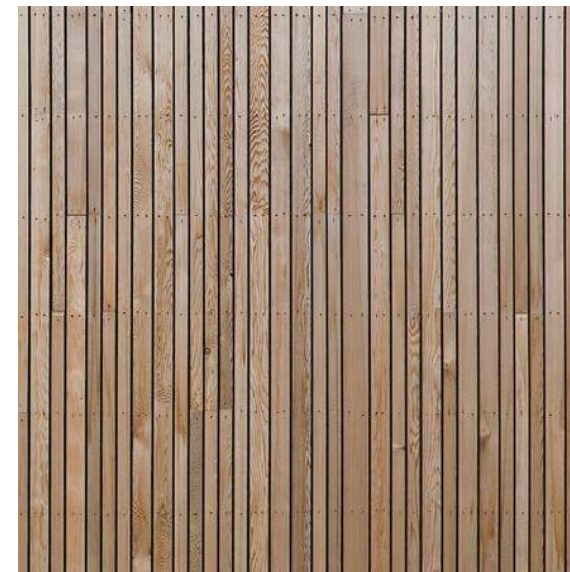
TMB1 - CLASS 1 SPOTTED GUM OR IRONBARK TIMBER BATTENS - CUTEK OIL FINISH OR SIMILAR
