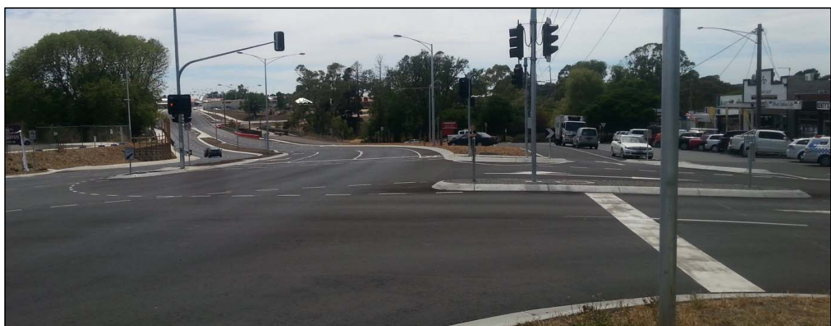
Figure 6: View of Main Street looking northeast from Hesse Street
