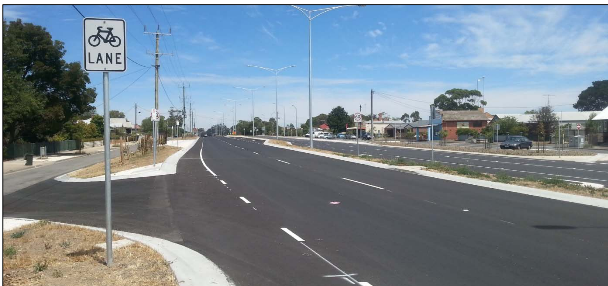
Figure 17: View of Princes Highway looking west from Hesse Street
